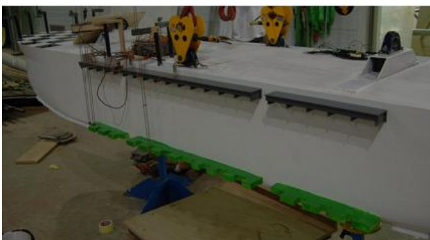
Figure 3: Lower and upper riser balcony on FPSO-1 (top) and FPSO-2 (bottom).
