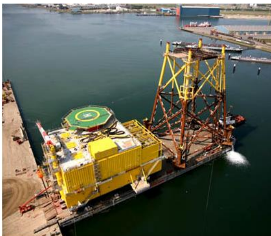
Figure 3: Transmission platform ready for tow out (courtesy Heerema Fabricators)
